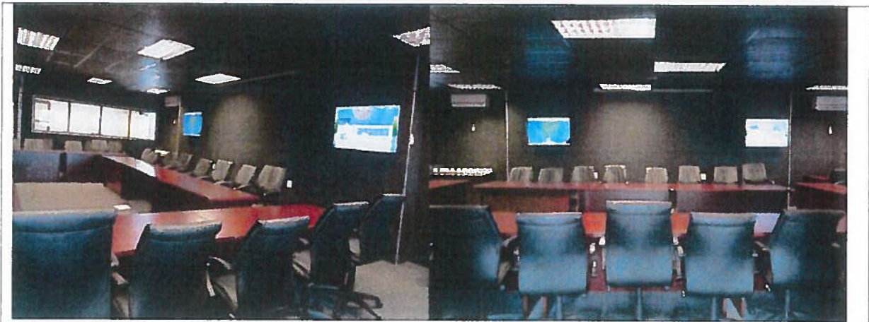
Figure 2: Main Boardroom – Operations Centre with displaying screens. The Operations Centre is used as a Disaster Operations Centre (DOC); Central Communications Centre; and Training, Media and Public Information Centre
