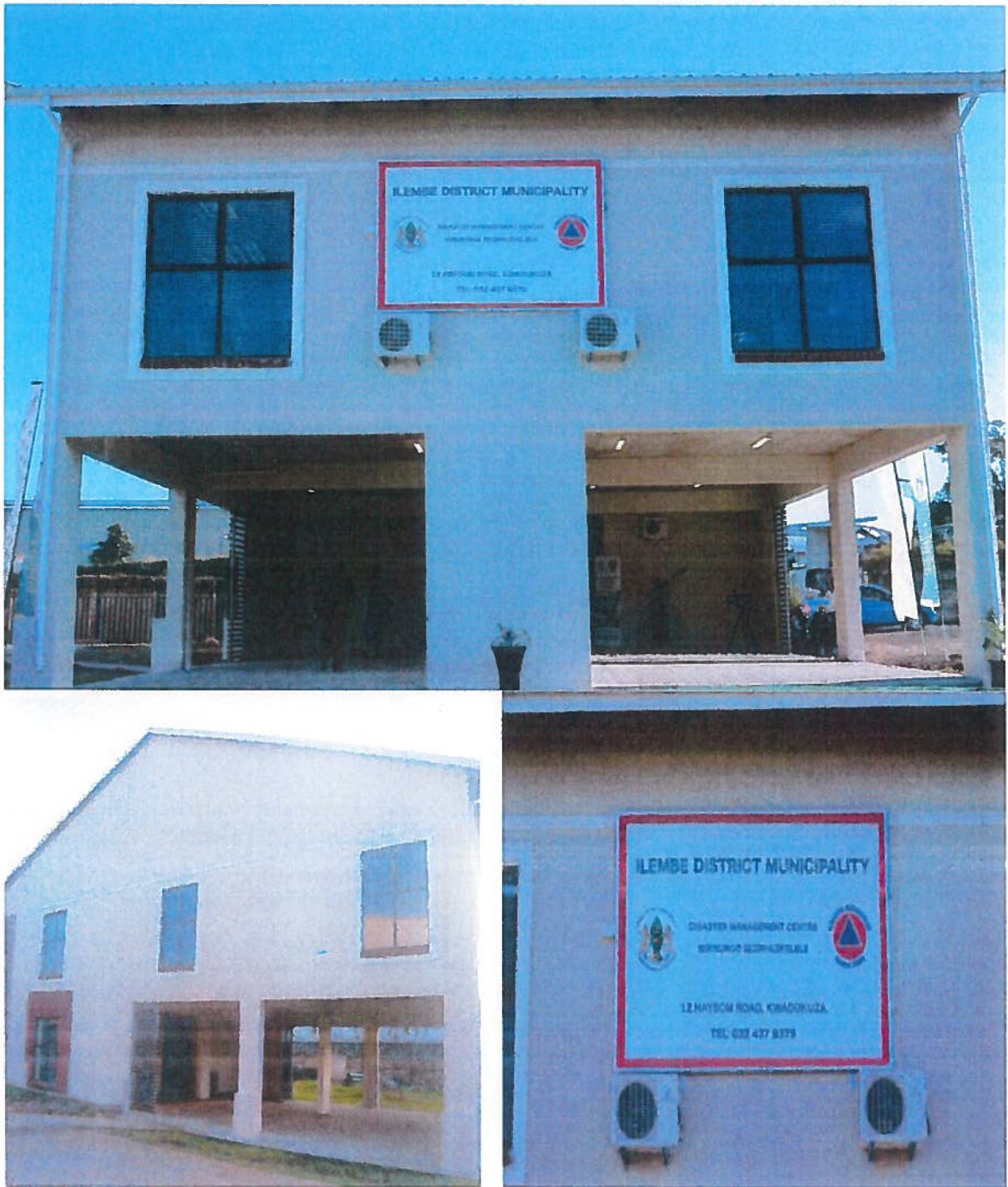
Figure 1: Pictures of the District Disaster Management Centre
